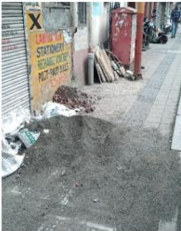
Photo 15 Construction material on footpath at Bajirao Road
